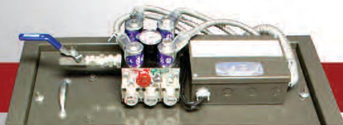
Close-Up of Reservoir Adjustment Valves
